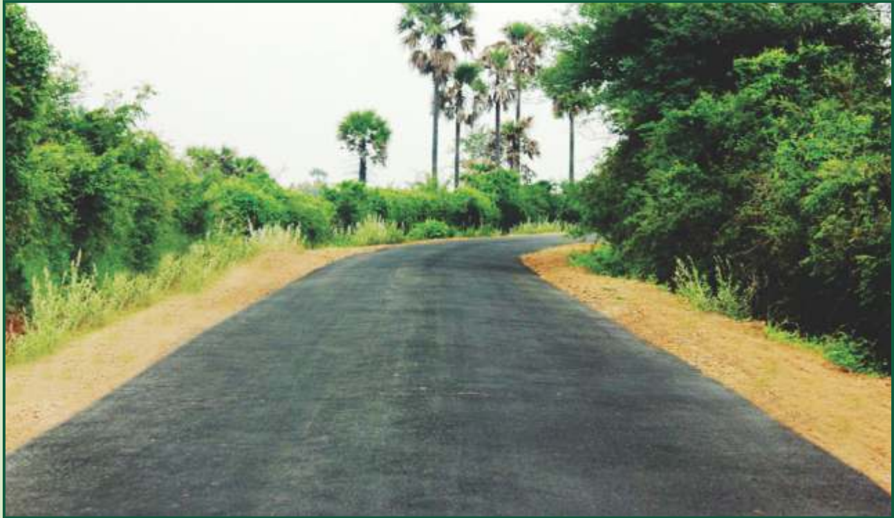
Formation and Black Topping of Road under NABARD - RIDF, Karur District
